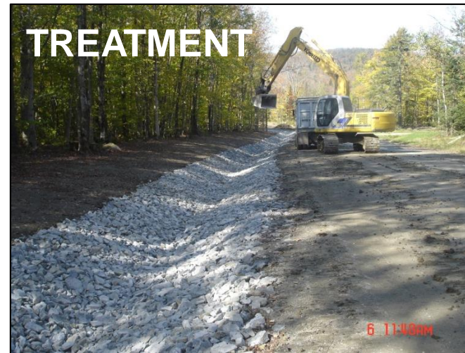
Ditch stabilization saves road and reduces erosion
